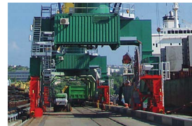
Traffic must also flow on narrow quays. The portal is built high enough to enable vehicles of all types to pass underneath it.
